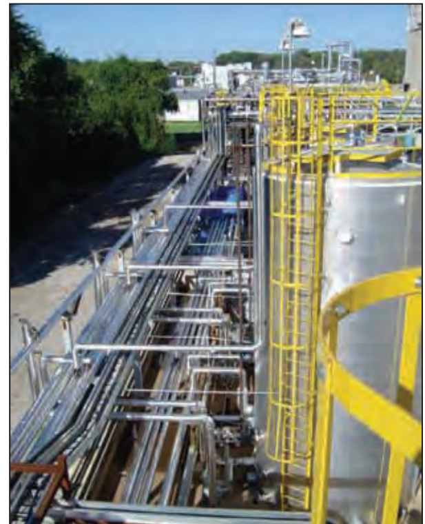
At the facility in Carthage, Missouri, the thermal depolymerization system developed by Changing World Technologies transforms ordinary poultry guts into diesel fuel.
