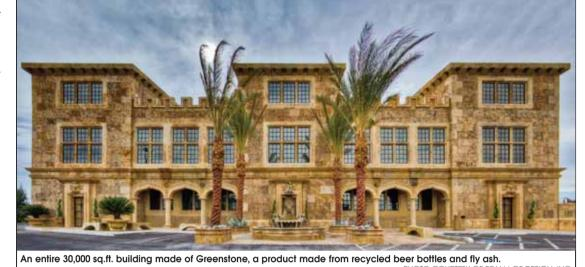
ash, a byproduct from coalfired power plants. Made in different colors, it can be poured into blocks, panels, or shaped in molds for whatever building material is required.
