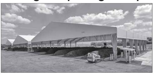
The Lee County Composting Facility (LCCF) in Felda, Florida, has constructed three new tension fabric buildings as part of an expansion project that will double the operation's production capacity for recycling biosolids and yard waste. The fabric structures were designed, manufactured and installed by Legacy Building Solutions.
