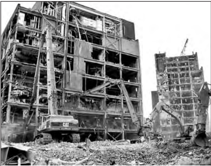
North American Dismantling Co. on location during a demolition job.
