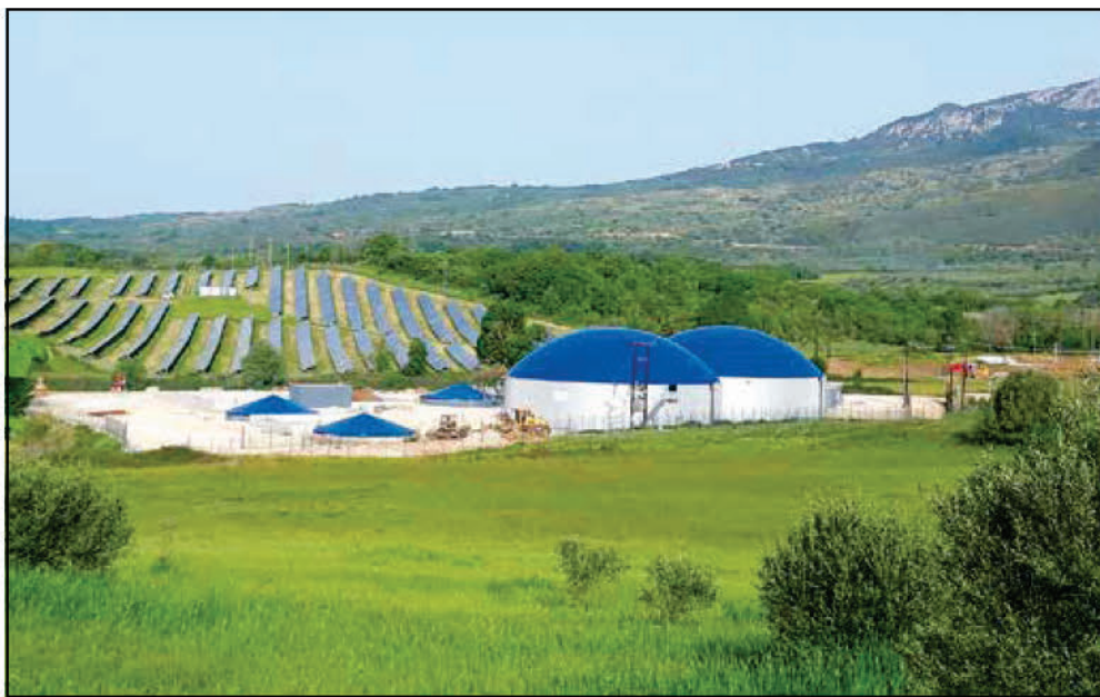
Weltec Biopower and Tetoros Machinery has built three biogas plants.
