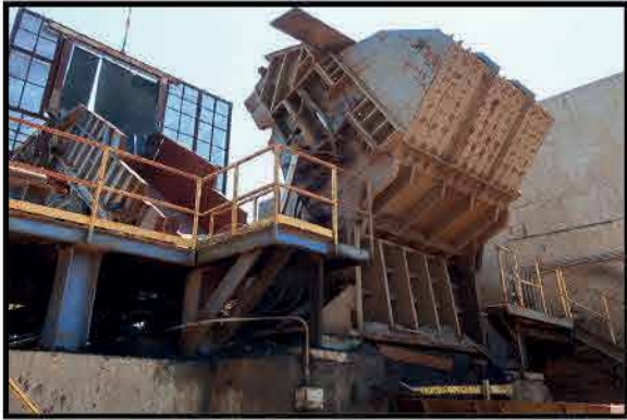
METSO TEXAS 80X104 HAMMERMILL SHREDDER INCLUDES FEED CHUTE, MILL, ROTOR, AND PIN PULLER
