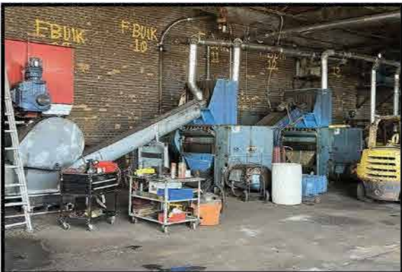
ELDAN TIRE RASPER SHREDDING / CRUMB LINE THREE ELDAN R-1200-1 RASPERS, MULTIPLE SCREENS, CONTROLS INCL.
